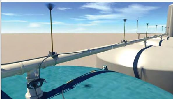
Dissipation Air Terminals Bonded with Class 1 Conductor on Fiberglass Pipe
