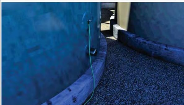
C Veil Bonding on Fiberglass Tank
