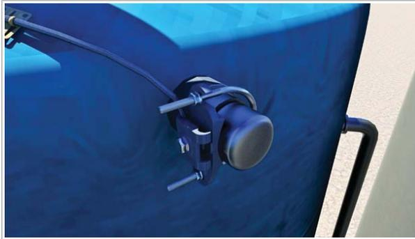
Metal Bull Plug on Fiberglass Tank Bonded with Class 1 Conductor
